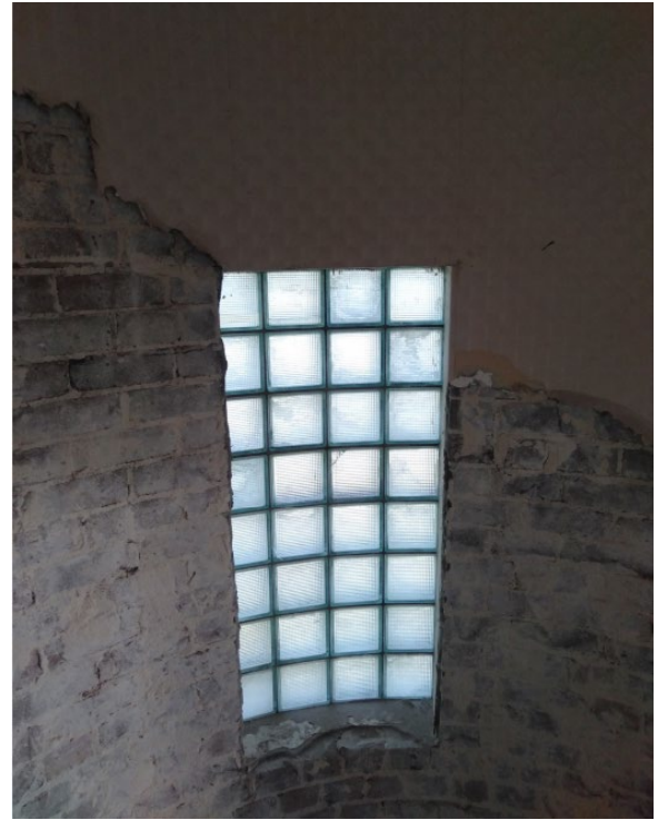
Figure 4.23 Glass block window in internal stairwell, also remnant wallpaper. (Source: GML, July 2024)
