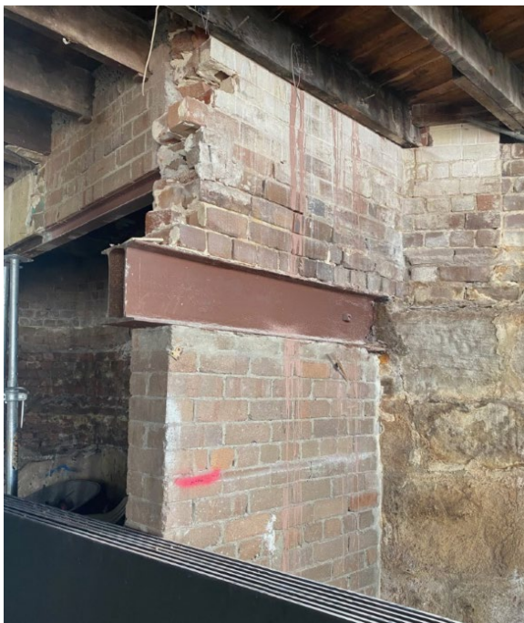
Figure 4.20 Severed beam in basement. (Source: GML, July 2024)
