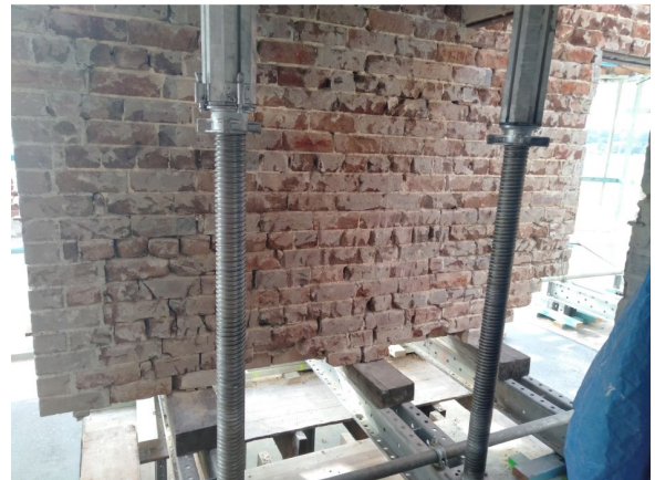
Figure 4.25 Section of wall partly removed, with temporary supports. (Source: GML, July 2024)
