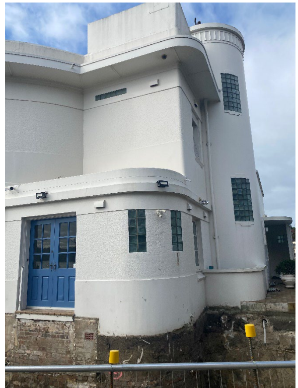
Figure 4.13 View of southwest corner, showing main entrance (stairs removed from excavation) and glass block windows on first floor curved elevations. (Source: GML, July 2024)
