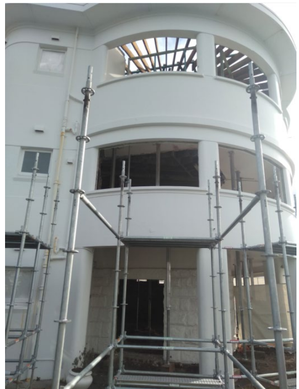
Figure 4.17 Eastern elevation of dwelling showing 1916 sandstone basement wall (painted white) and form of 1939 addition above. (Source: GML, July 2024)
